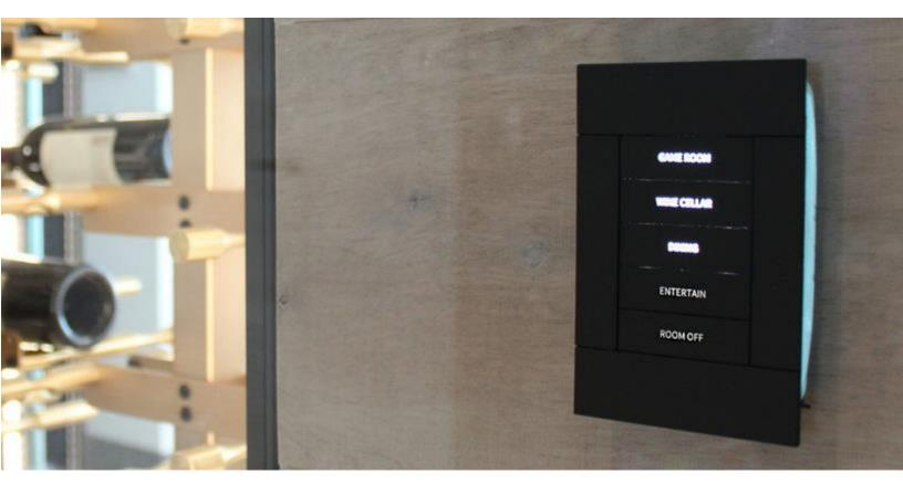
Also known as the "Centralized Lighting System" or the "Integrated Lighting". It is called centralized because it is powered by wall wiring that leads to a single processor.
